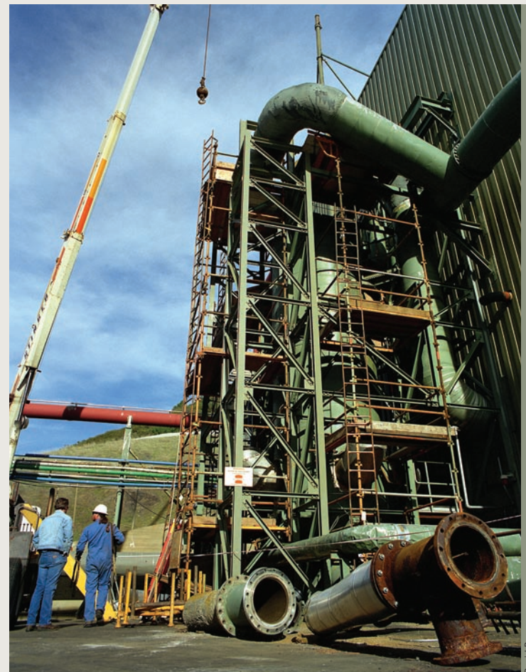
Condensers being retrofitted with direct contact condensers at The Geysers Geothermal Power Plant in California.
