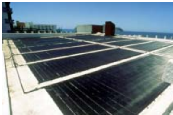
A solar heating system requires very little or no maintenance since it has no burners or moving parts. NREL/PIX08590
