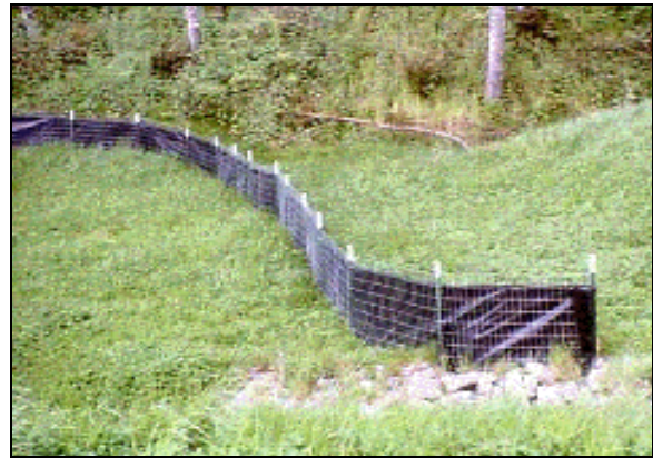
Silt fencing helps to avoid construction delays and work stoppages due to erosion. NREL/PIX 11409
