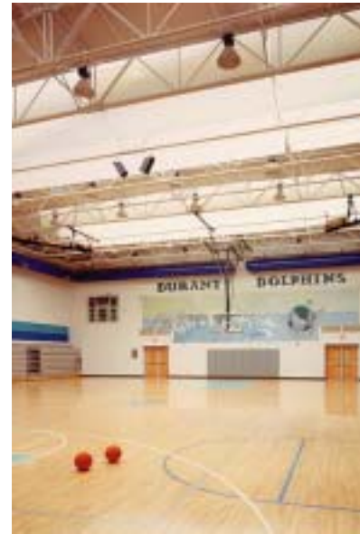
Monitors provide diffuse light into gymnasiums. NREL/PIX 11338
