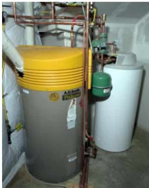
This central, high-efficiency boiler supplies hot water to two insulated storage tanks, providing hot water to six baths and a radiant floor heating system. NREL/PIX07925
