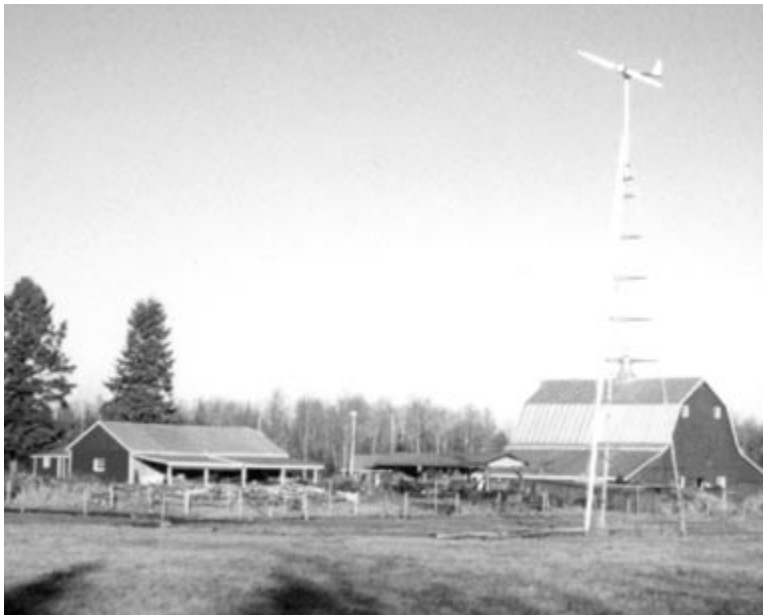
In Clover Valley, Minnesota, this 3-kW Whisper H175 turbine on a 50-foot tower is connected to the utility grid to offset the farm's utility-supplied electricity.
