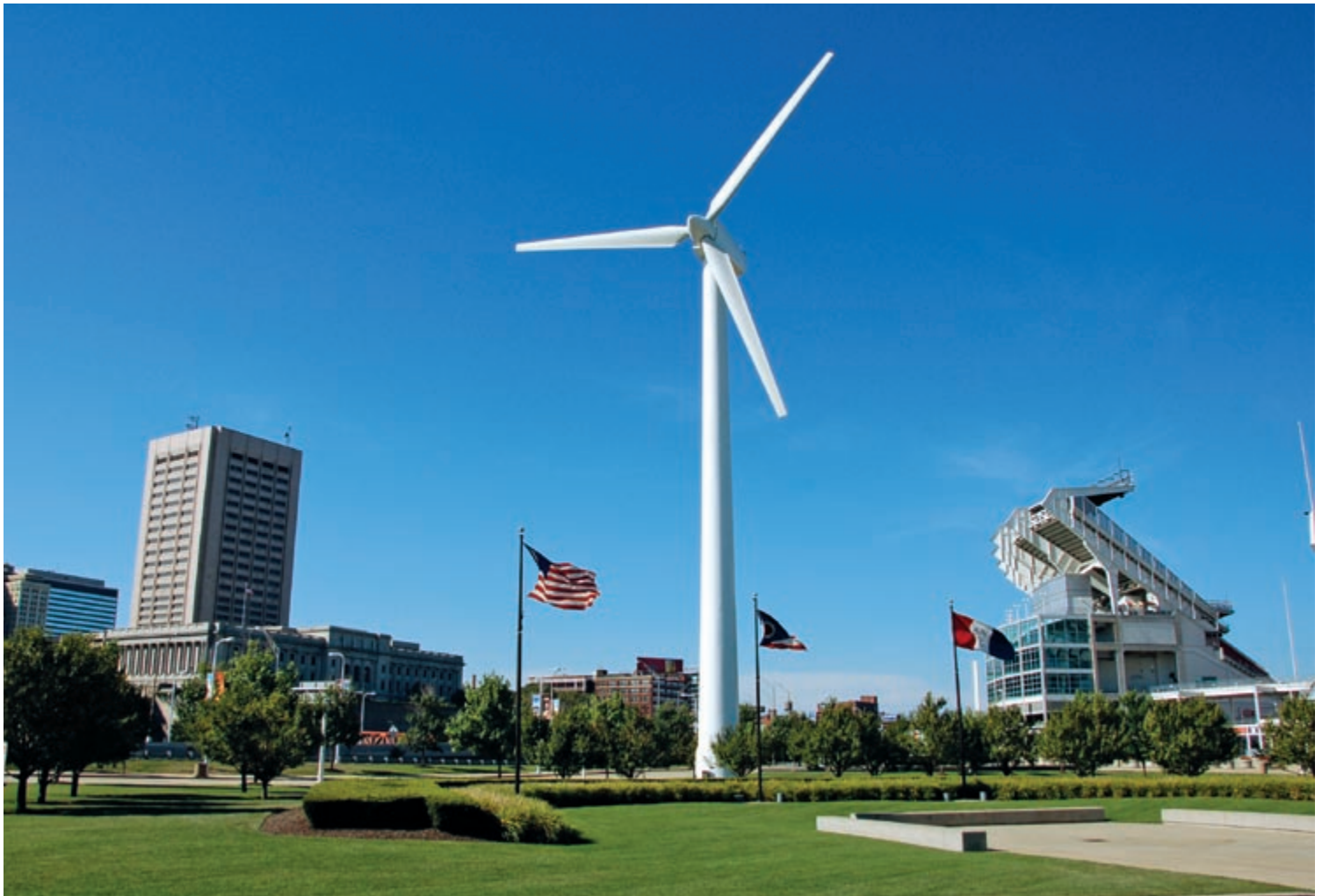
The Ohio Wind Working Group (OWWG) assisted with the installation of an educational, utility-scale Vestas 225-kW wind turbine in downtown Cleveland, located directly in front of the Great Lakes Science Center and next to the Rock & Roll Hall of Fame and the Cleveland Browns Stadium. Photo credit: Tom Maves/ PIX14827
