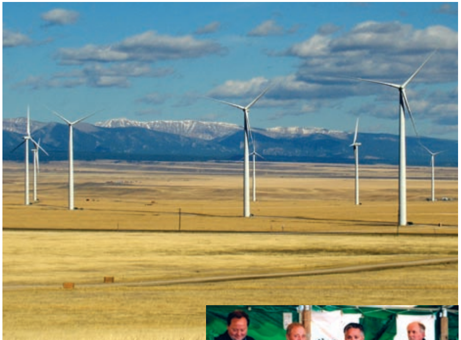
The Judith Gap Wind Energy Center in Montana is comprised of 90 GE 1.5-MW turbines, for a total capacity of 135 MW. Photo credit: Invenergy LLC/ PIX14371
