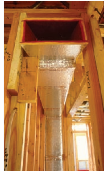
Properly sized and sealed ducts, kept inside conditioned space, improve performance and reduce cost. Source: IBACOS
