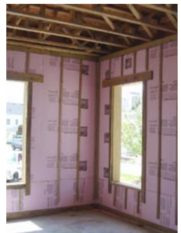
FIGURE 11: Masonry Walls with Interior Rigid Insulation
