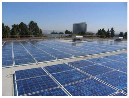
Figure 55: Demonstration array with reduced coating thickness during installation
