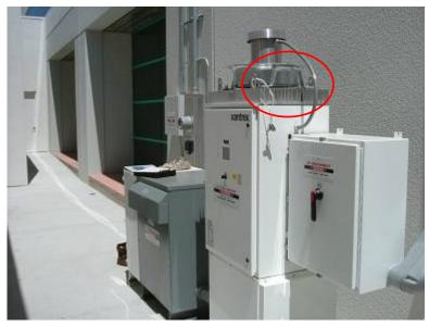
Figure 7: Xantrex S-Series inverter installation with PowerLight DAS
