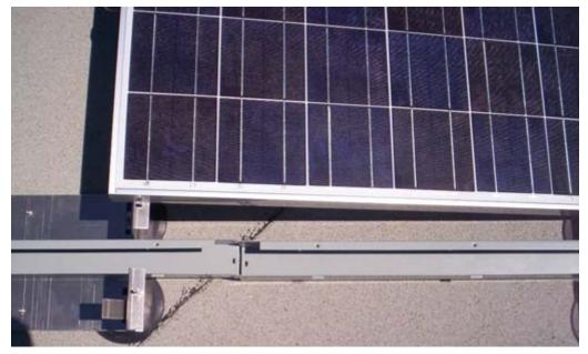
Figure 57: Wiring gutter during installation (designed changed after this installation)
