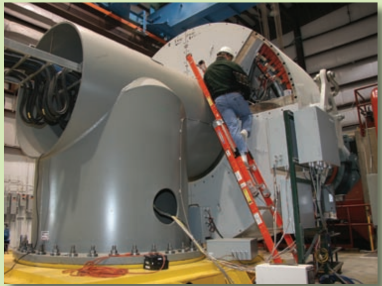
The NPS 1.5-MW permanent-magnet direct-drive prototype generator tested at NREL.
