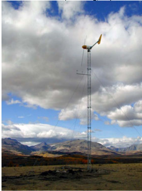
Photo 4: Turbine installed at Nelson farm Source: NWSEED
