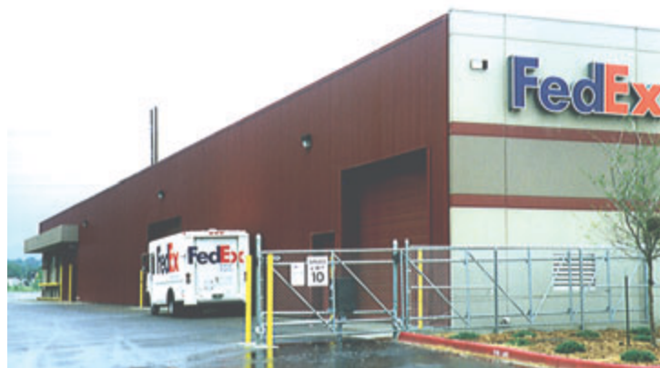
Transpired air collector ventilation preheating technology is ideal for sunny locations with long heating seasons, such as for this Federal Express facility in Colorado.
