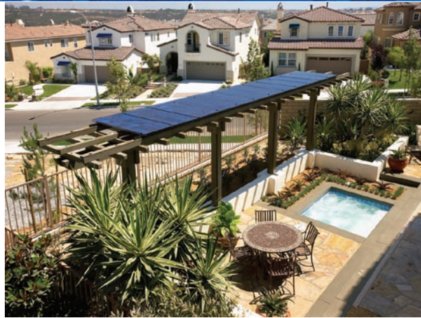
This home features an attractive solar trellis next to the rear courtyard oasis. Built by Pardee Homes of San Diego, California, the home was a 2005 EnergyValue Housing Award gold winner in the Production Home, Moderate Climate category. All homes in this subdivision are highly efficient and have 2.4-kW PV systems. Credit: NAHB Research Center
