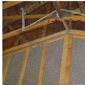
Blown-in wall insulation
