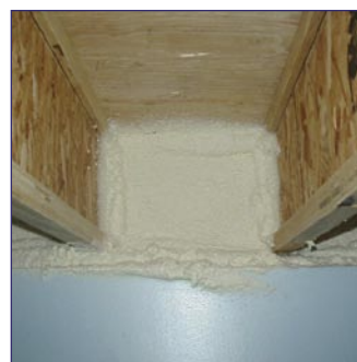
Soy-based foams are now available (Photo: Building Science Corporation)
