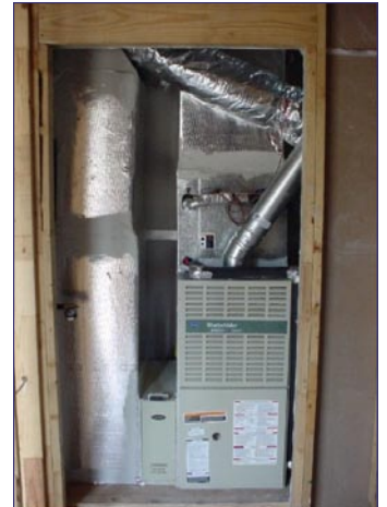
A fresh air intake duct with a Constant Airflow Regulator runs from the outside to the return plenum. The furnace operates continuously on low speed to provide whole-house ventilation.
