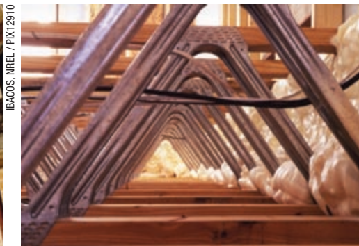
Open web trusses provide space within the building enclosure to run electrical wires and ducts.
