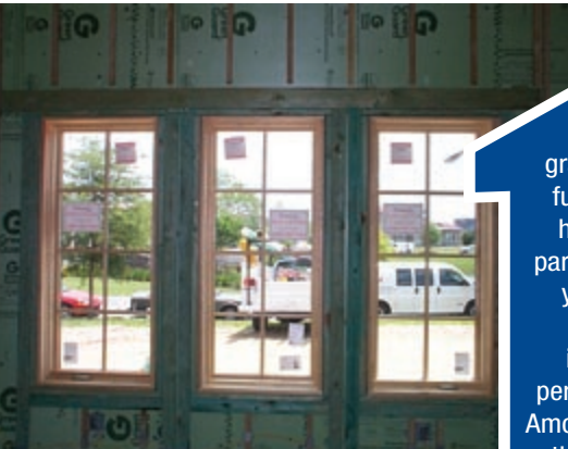
Low-emissivity windows help to save energy on heating and cooling the home.
