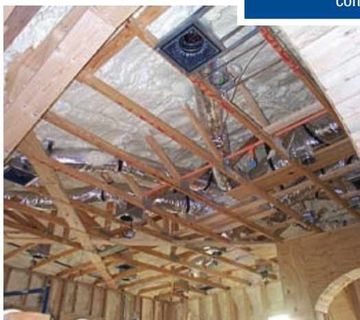
Spray foam insulation keeps the ductwork within conditioned space.
