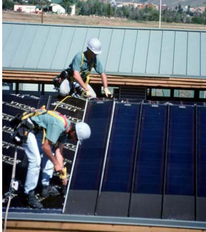
Figure 5-9 Installation of the roof-integrated PV panels
