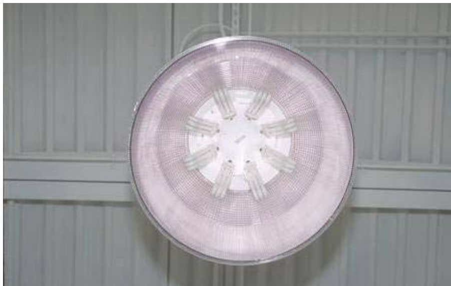
Figure 5-7 Pendant luminaire with eight 42-Watt CFL bulbs used in the retail and warehouse areas
