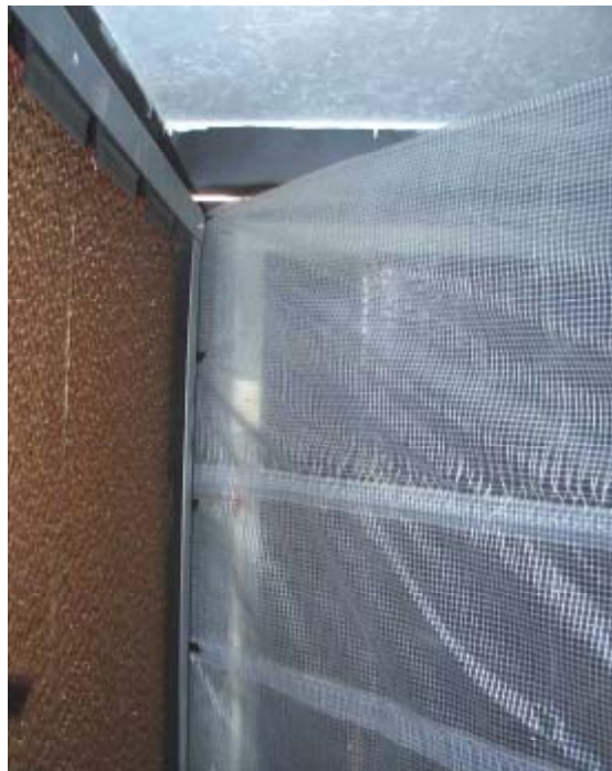
Figure 6-10 Plastic blocking device for cooltowers
