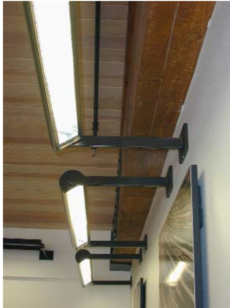
Figure 4-6 Display lighting using 4-ft T-8 Lamps
