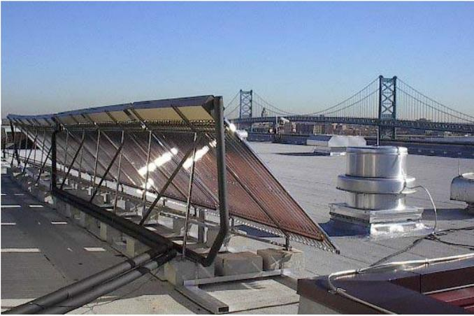
**Figure 1. Photograph of the solar array on the southwest riser of the building recirculation loop on the Mid-Atlantic Social Security Center, Philadelphia, PA; another array on the northeast riser is identical in size and orientation.**
