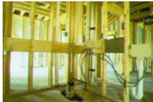
Fig. 10: Installing blocking in walls around tubs and toilets provides the structural support for the installation of grab bars.
