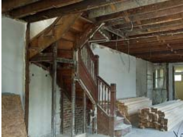
Fig. 2: To save on costs, the original stairway was maintained.
