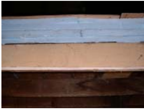
Fig. 27: 4 layers of 2" rigid insulation (Total R=40) installed on the attic floor. Joints between insulation boards should be staggered.
