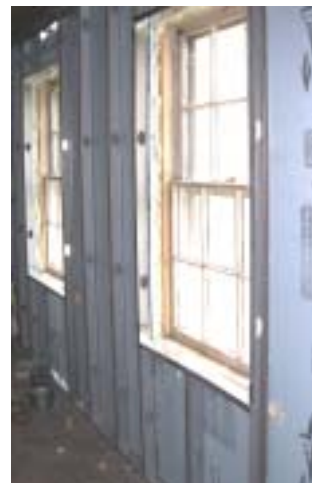
Fig. 25: Sealing joints between rigid insulation boards
