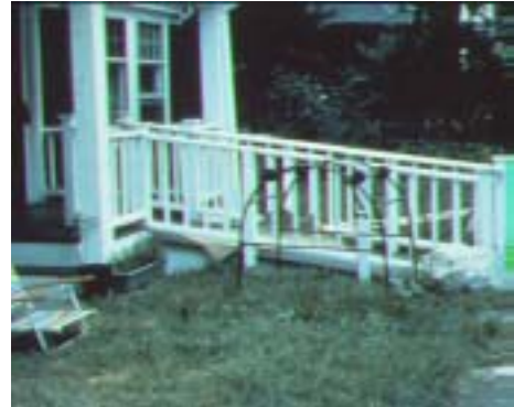
Fig. 11: An accessible entrance makes this home “visitable.”
