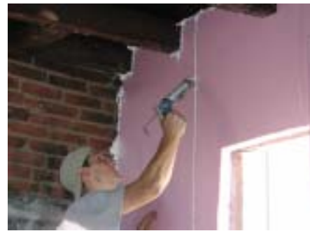
Fig. 25: Sealing joints between rigid insulation boards
