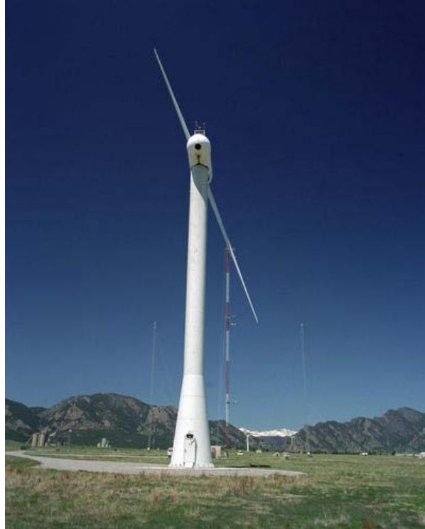
Figure 3-1. NWTC inflow measurement array upwind of ART, looking toward prevailing wind direction
