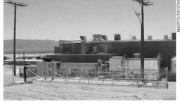
A 7-MW cogeneration system is part of a comprehensive set of energy and facility upgrades at this Marine base in Twentynine Palms, California.
