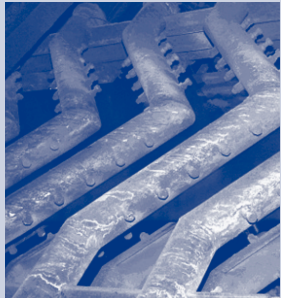
Hot-Air Strip Dryers for a Continuous Annealing Line (Project 2)
