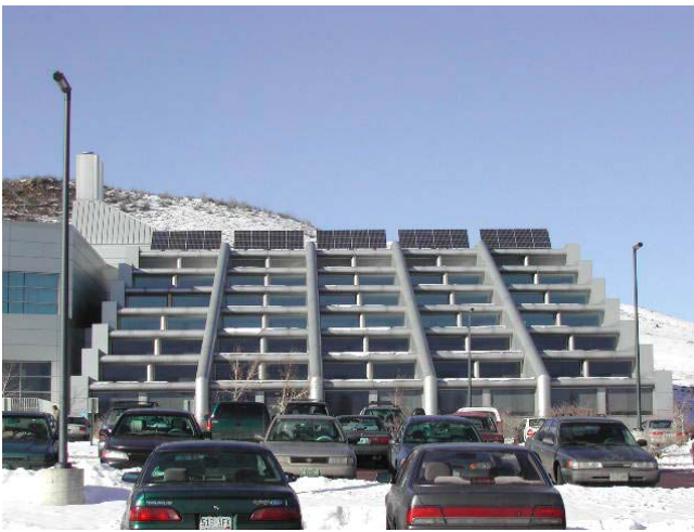
Figure 1. SERFEAST array on the roof of the building.
