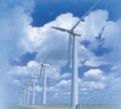
*This wind farm in southeastern Wyoming contains 69 600-kW wind turbines that provide green power for the customers of Eugene Water and Electric in Eugene, Oregon. Each turbine has a hub height of 130 feet, three 66-foot blades, and weighs approximately 30,000 pounds.*
