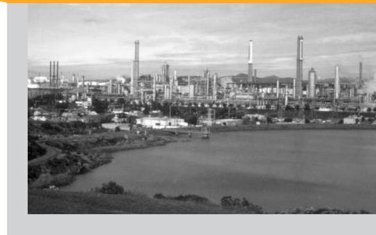
The refinery processes primarily San Joaquin Valley crude oil at the rate of 165,000 barrels of oil per day. It is a high-conversion refinery comprising catalytic cracking, hydrocracking, and coking operations as well as the basic distillation and catalytic reforming processes. The plant includes lubricants and asphalt facilities. Energy costs for the facility were approxi-
