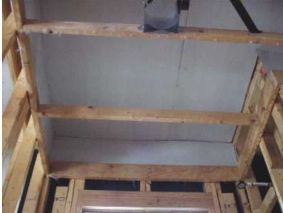
Figure 11. Draftstopping applied at the top of the second-floor bulkhead.
