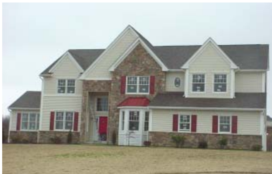
Figure 12. Front of pilot home with Owens Corning cultured stone and vinyl siding.
