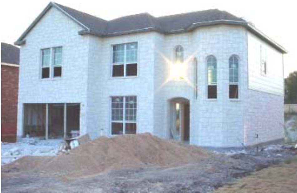
Figure 8. Front elevation of the pilot home with synthetic stone cladding.
