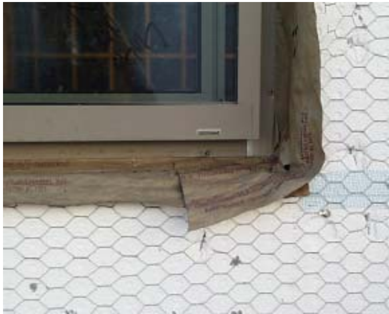
Figure 20. Windows are flashed with an adhesive membrane.
