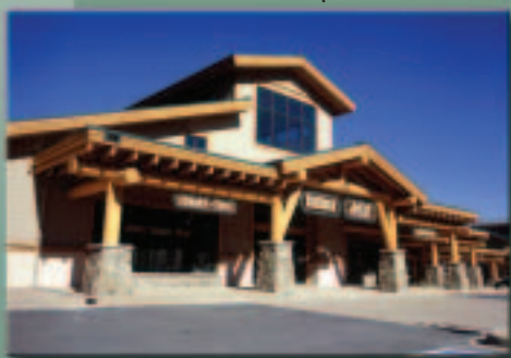
The BigHorn high-performance building features PV, clerestory windows, daylighting, diffusing skylights, and solar wall. Anticipated energy cost savings from all the features, not including PV, is 62%.
