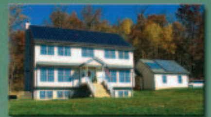
The "Solar Patriot," in Virginia has a 6-kW PV system, solar water heater, geothermal heat pump, compact fluorescent lighting, high-efficiency appliances, and low-e windows.
