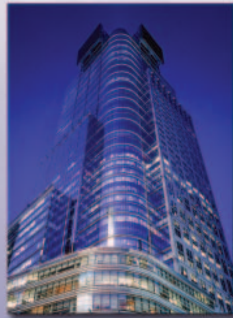
The 4 Times Square building in Manhattan uses thin-film PV panels to supply 15 kW of power to supplement the building’s electricity needs. Located on the top 14 floors on the south and east sides of the building, the PV panels are integrated into the spandrel—the opaque area of the façade below rows of windows—in 60-inch-wide strips. (Andrew Gordon Photography.)
