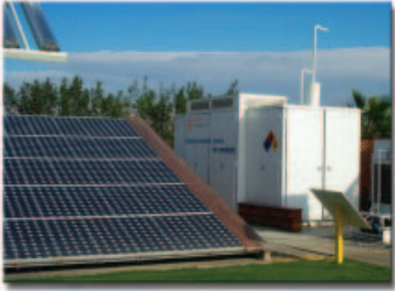
This photovoltaic system at SunLine Transit Agency in Thousand Palms, California, provides electricity for the Stuart Energy electrolysis unit (on the right).
