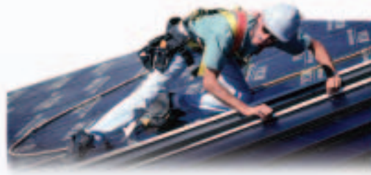
Installation of PV-integrated standing-seam metal roof panels.
