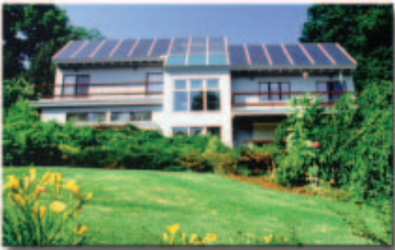
The Impact 2000 home in Massachusetts uses a 4.5-kW utility-interactive PV system. It also incorporates many other energy efficiency and renewable energy features—solar hot water, super insulation, passive solar heating and cooling, and an earth-coupled, geothermal heat pump.
