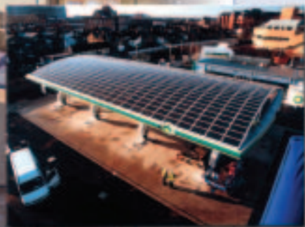
BP Solar's new semi-transparent amorphous silicon modules—developed through participation in the Amorphous Silicon National Research Team—are used to provide power to run pumps, lights, and other loads at BP gasoline stations.
