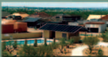
The pool of the Civano development in Tucson, Arizona, uses a 6-kW photovoltaic installation to help meet the community’s energy standard.
