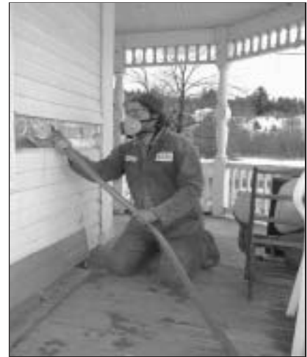
Technicians install dense-pack insulation to reduce heat loss and air infiltration.
