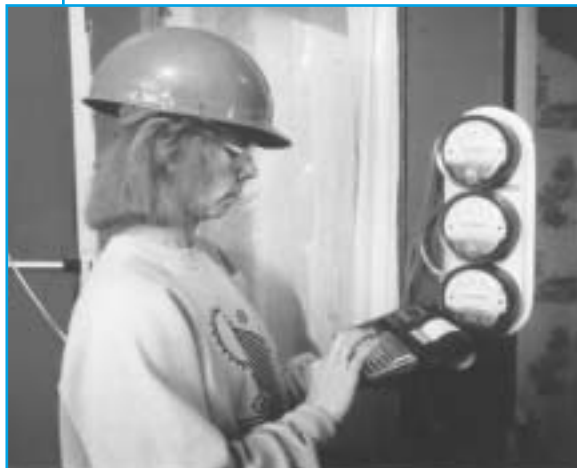
Weatherization technicians utilize blower door technology to diagnose and mitigate air infiltration.
