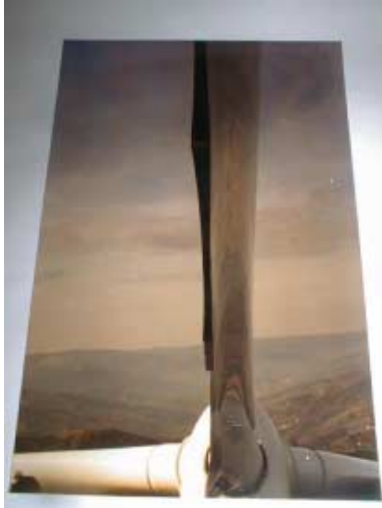
Figure 7. IVPC/Vestas blade damage
