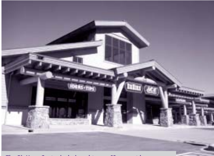
The BigHorn Center is designed to use 62 percent less energy than a conventional building.
