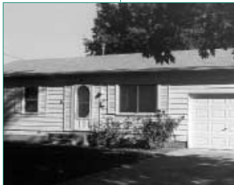
Macomb County Community Services Agency leveraged funding and partnered with “Paint the Town, Inc.” to perform extensive weatherization and renovation work for this low-income home.
