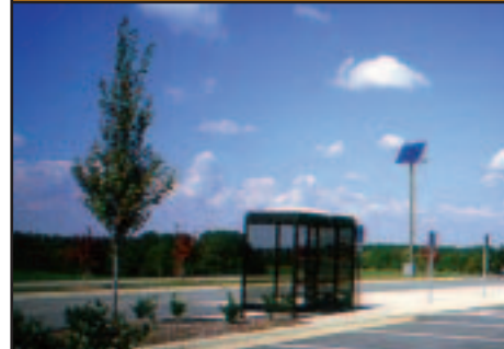
These stand-alone photovoltaic systems power parking lights.
