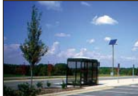
These stand-alone photovoltaic systems power parking lights.
