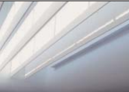
Translucent baffles block direct beam radiation and diffuse the sunlight throughout the space.
