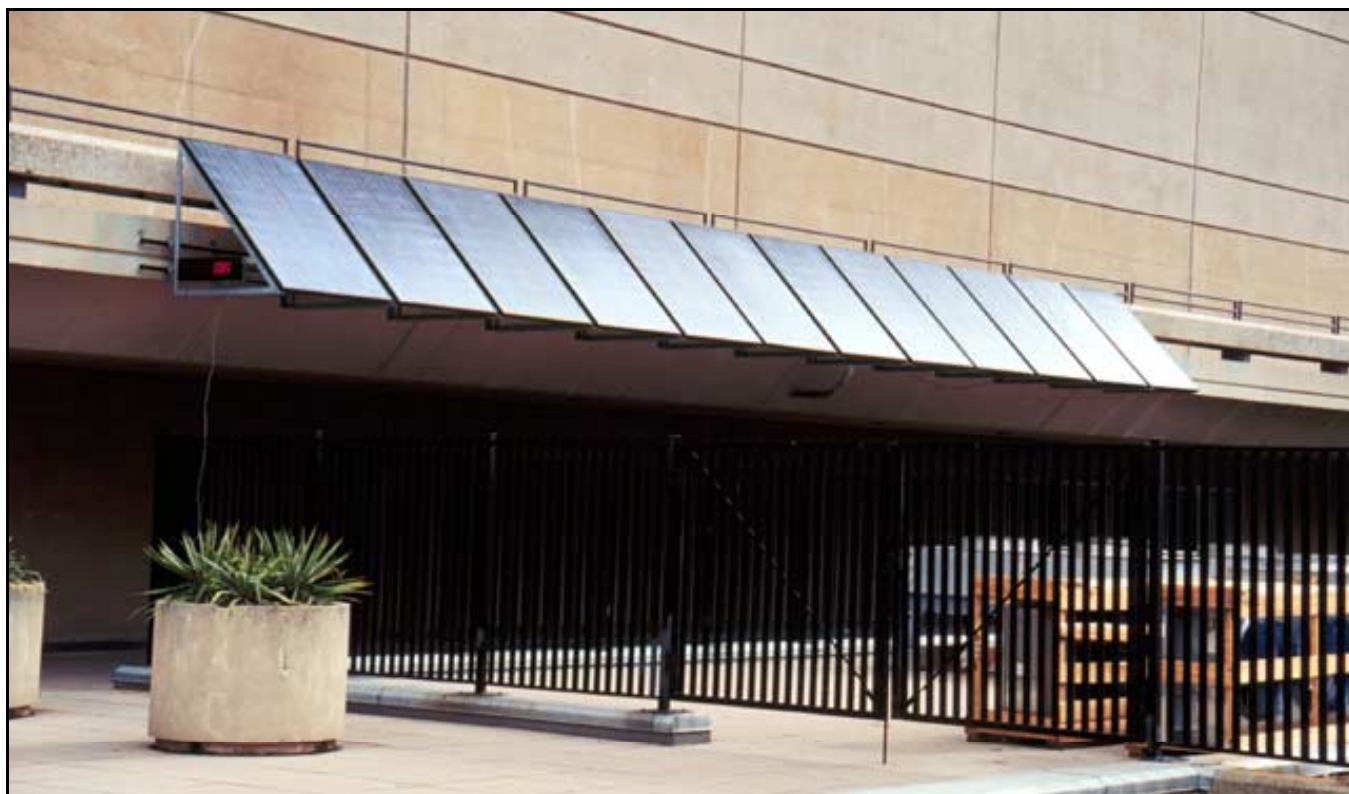
Figure 2. View of U.S. Department of Energy's cantilevered PV system on the Forrestal Building. (Photo: B. Stafford)
