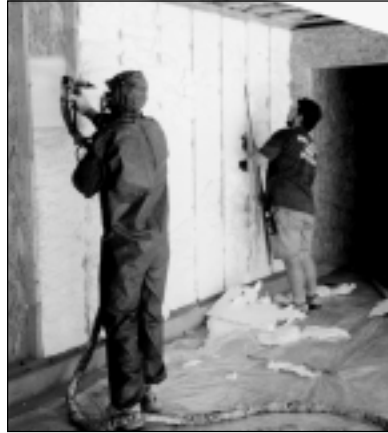
Figure 31. Spray foam insulation.
