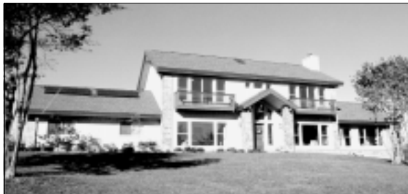
Figure 14 and 15. Passive solar homes can be both attractive and traditional in appearance. These two attractive solar homes take full advantage of solar heat gain and shading to minimize unwanted heat gain during the summer months.
