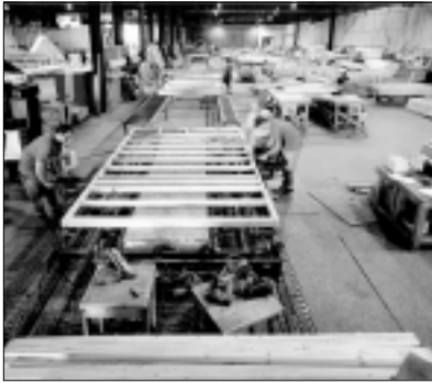
Figure 26. Prefabricated wall sections are assembled in the factory for shipment to the construction site.
