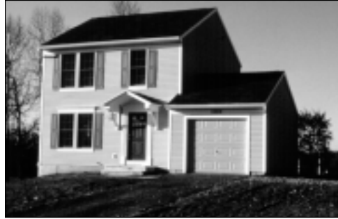
Figure 47. This prototype house by NVR Homes proved that production builders can cost effectively implement energy- and resource-efficiency measures. NVR Homes puts a standard energy package in all of its homes.
