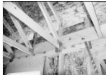
Figure 27. Raised-heel roof truss.
