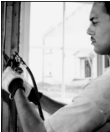
Figure 51. Air sealing around window openings.
