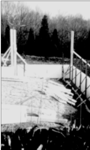
Figure 21. Insulating Concrete Form foundation under construction.
