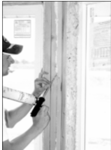
Figure 49. Air sealing around window openings.
