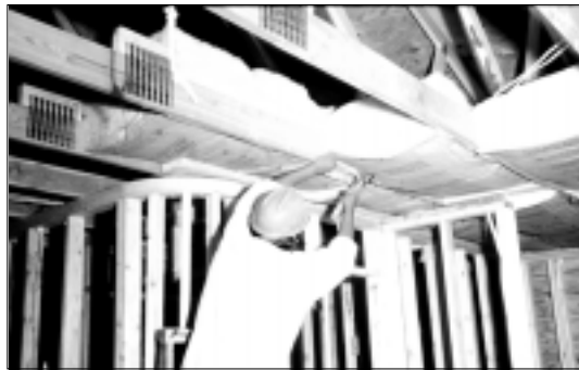
Figure 29. Batt insulation.
