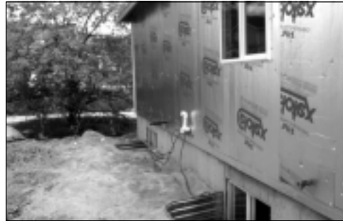
Figure 32. Insulating sheathing.
