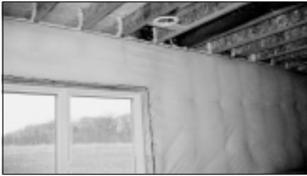
Figure 49. Rim joist detailing.
