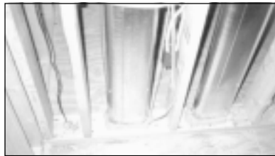
Figure 50. Air sealing ductwork penetrations between conditioned and unconditioned space.
