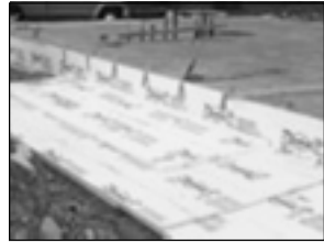
Figure 33. Frost-protected shallow foundation.
