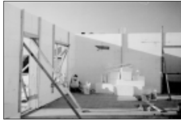
Figure 22. Insulating Concrete Form walls under construction.
