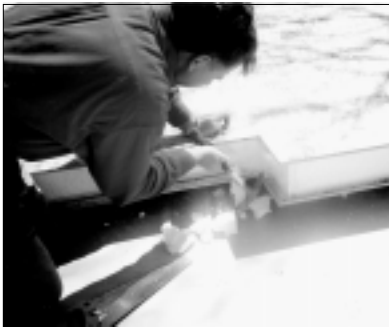
Figure 19. A worker cuts a Structural Insulated Panel to size.
