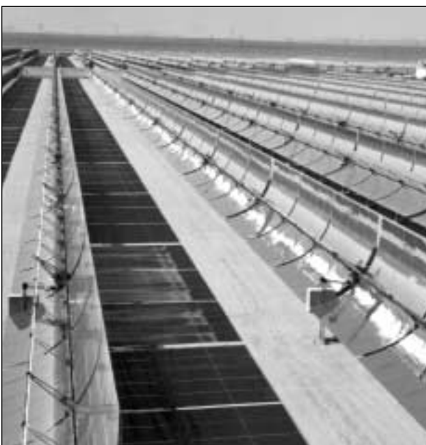
Nine trough power plants in southern California, with a capacity of 354 MW, meet the energy needs of 350,000 people.
