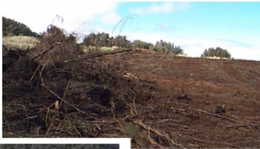
(b) Field during preparation.
