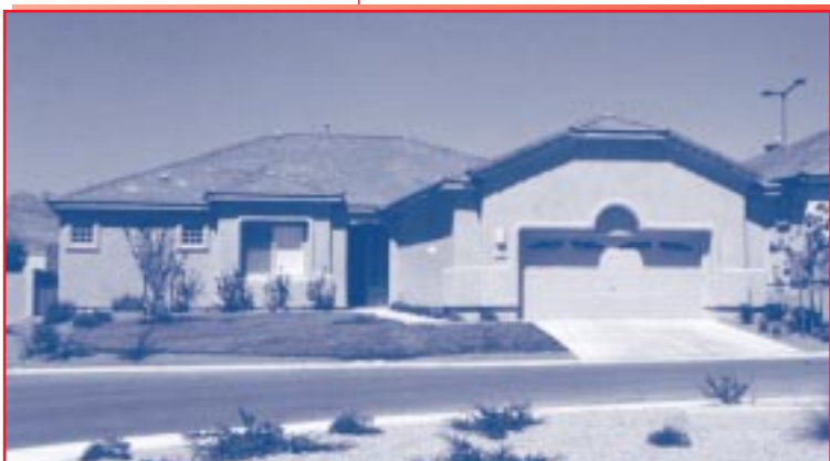
This Building America house built by Pulte Homes in Las Vegas meets Energy Star requirements and features an unvented roof, spectrally selective windows, and mechanical ventilation.
