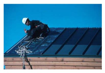
Figure 5. Installation of the Photovoltaic Roof
