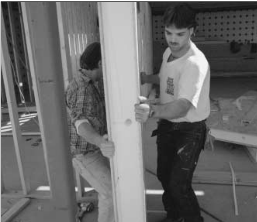
Workers install a structural insulated panel.
