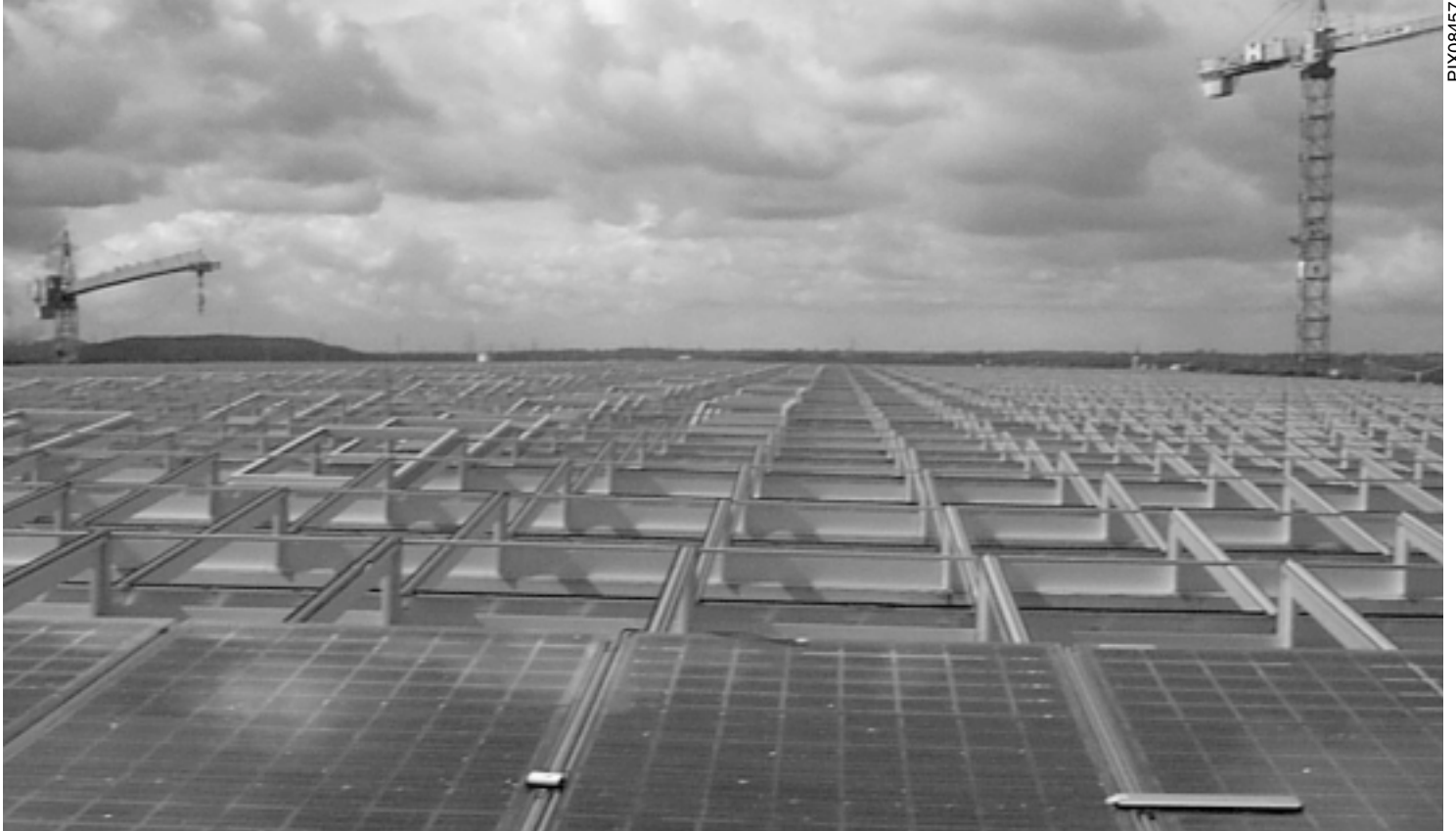
Rooftop view shows placement of insulation and PV panels.
