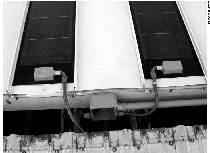
Additional electrical junction boxes were required over potted terminals and raceways at the ridge, before the ridge cap was installed.
