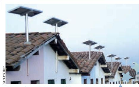
50-watt photovoltaic electric lighting systems provide four to six hours of light each night for residents of this village in Ceara, Brazil.
