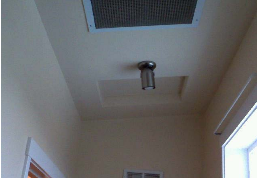
Upstairs attic hatch.
