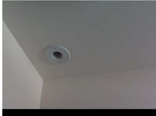
Air leakage from the roof penetration through the edge of the high velocity duct system
