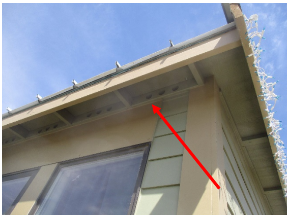
Soffit venting
