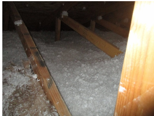
Upstairs attic insulation
