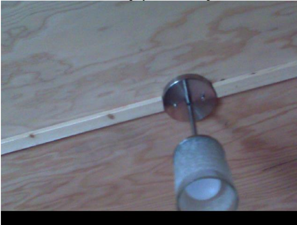
Light fixture in the wooden ceiling.
