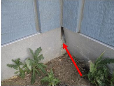
Left: Rigid Insulation has been pushed under the home, suggest replacing. Right: Conditioned Crawl space.
