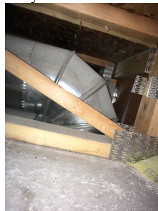
Left: Failed air barrier. This piece of plastic should be replaced with rigid form or some other more robust material. Right: Return air pathway.
