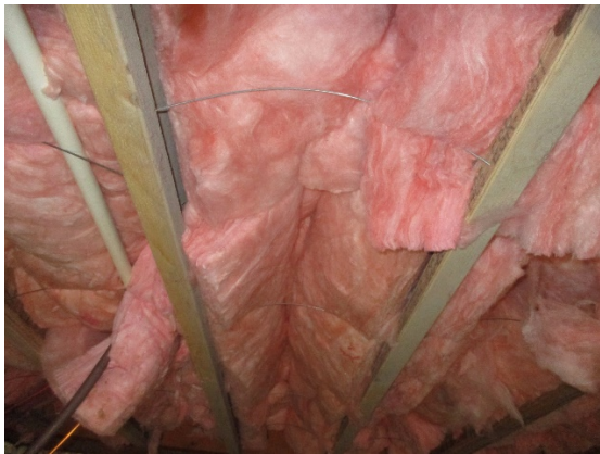
Crawl space insulation
