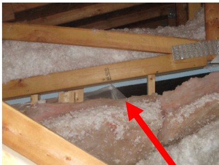
Left: Failed air barrier. This piece of plastic should be replaced with rigid form or some other more robust material. Right: Return air pathway.
