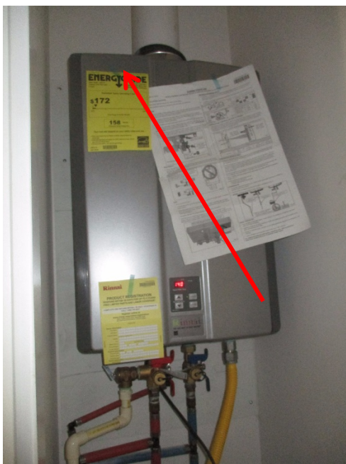
The combustion air supply should be connected at this location
