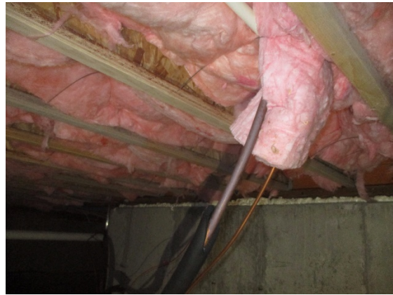
Main water line in the vented crawl space
