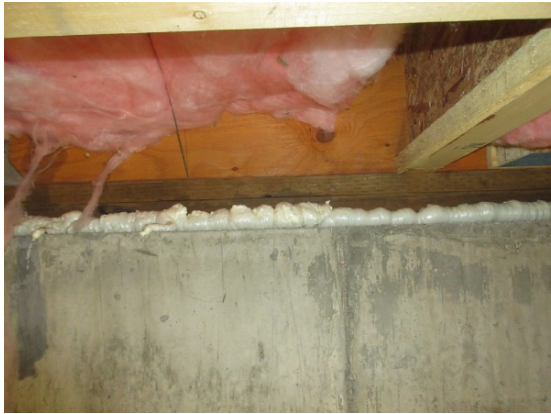
Additional pictures of the crawl space
