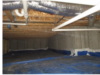
Left: Rigid Insulation has been pushed under the home, suggest replacing. Right: Conditioned Crawl space.
