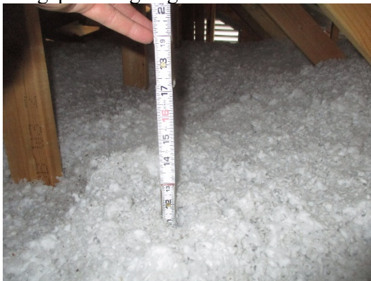
Depth of attic insulation 10"
