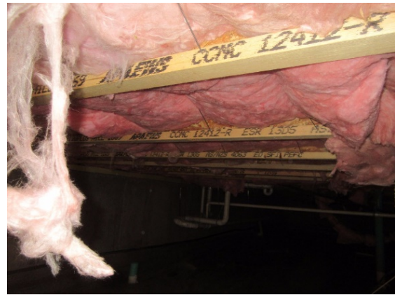
Compressed fiberglass batts
