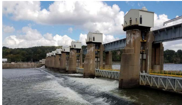
Figure 22. Emsworth Lock and Dam near downtown Pittsburgh, Pennsylvania—an NPD that Rye plans to retrofit to add 20 MW in generation capacity. Photo from Rye Development (2023)
