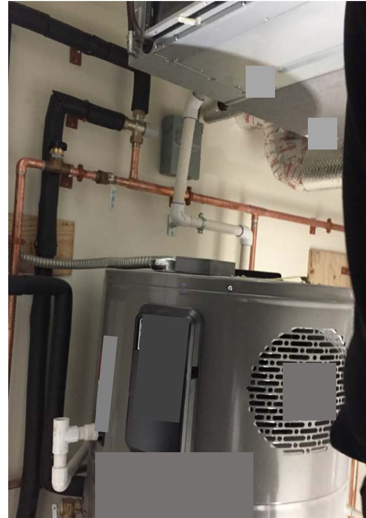
Careful planning around plumbing & electric.
