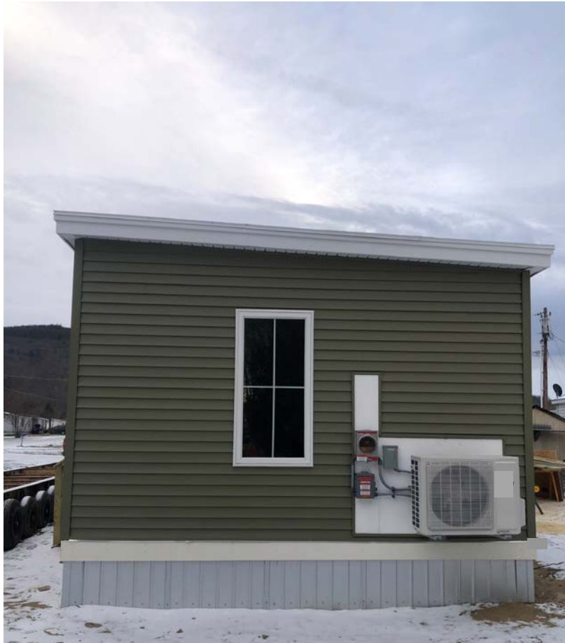
House delivered and set with HVAC already commissioned at factory.
