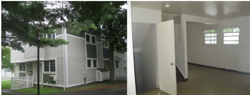
Figure 14. Typical NHA housing unit
