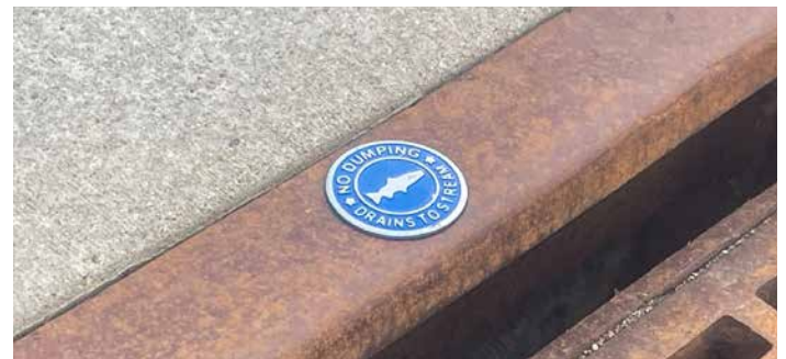
Placard discs were applied to the stormwater drains on NREL's South Table Mountain Campus as a part of the MS4 permit program.
