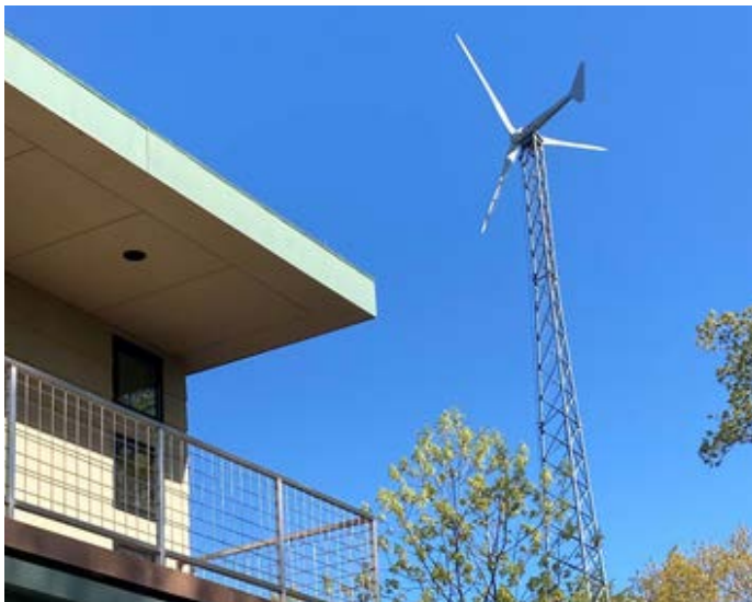
A Bergey Excel 15 wind turbine installed at a residence in Avon, Connecticut. Photo from Mike Bergey, Bergey Windpower
