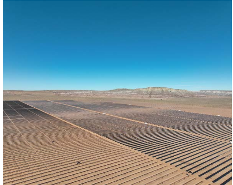
Aerial view of the NTUA Red Mesa array
