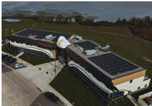
70-kW rooftop array at the Red Lake Band's Tribal government center
