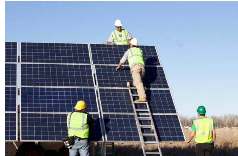
Installing one of the five solar photovoltaic projects
