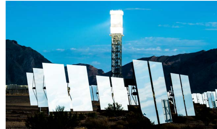
Figure. Concentrating solar-thermal power plant
