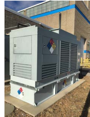
Example of Backup Diesel Generator
