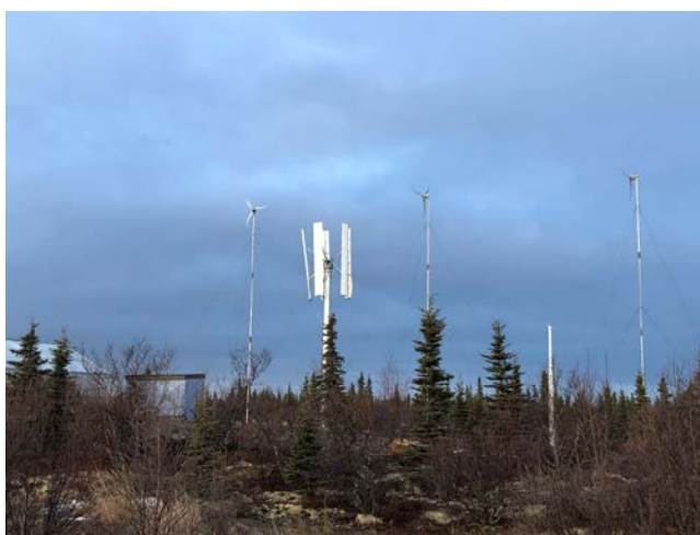
Figure 2. Several small wind turbines are installed near the Igiugig village greenhouse, with Skystreams visible in the distance and a vertical-axis wind turbine in the foreground. Photo by Rebecca Green, NREL
