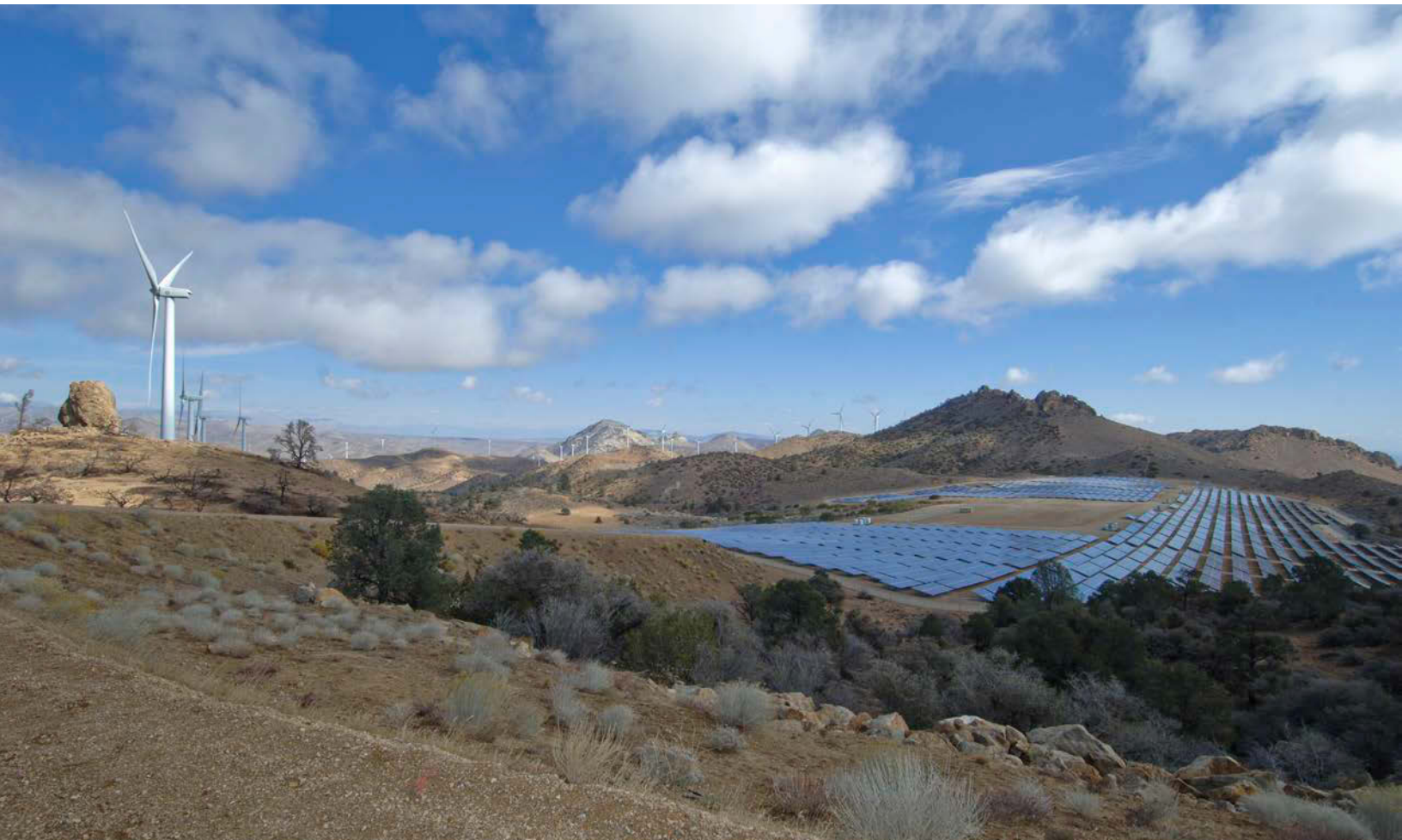
LADWP's Pine Tree Wind and Solar Farm. Photo from LADWP
